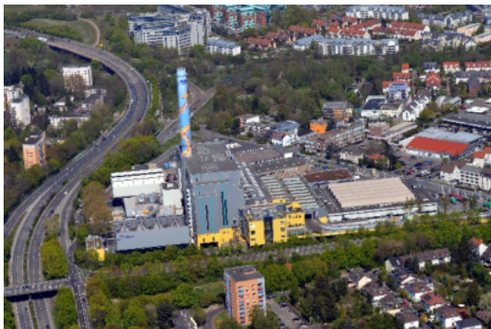
MHKW Frankfurt am Main
