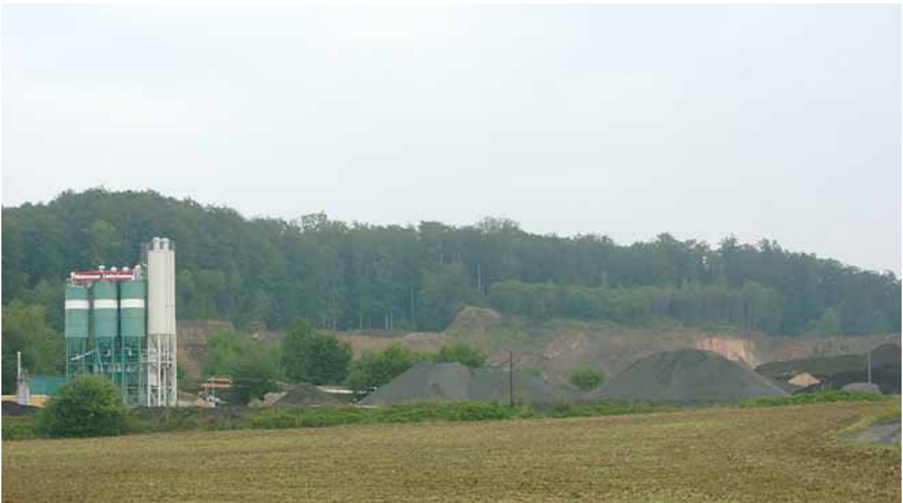
Basaltsteinbruch Eltersberg in Alten-Buseck
